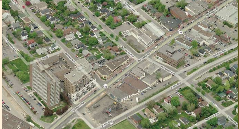
Obsolete giving way to inner city intensification. Source: Bing Maps
